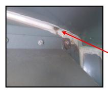
If a leak has occurred a visual check will show a clean area on the bin wall that is usually dusty. This is caused by an air stream coming through the bin divider and blowing product from a section of the wall around the leak area.
